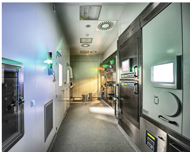
Figure 4. Hot cells in the Research Laboratory [photos: Grzegorz Krzyżewski]
